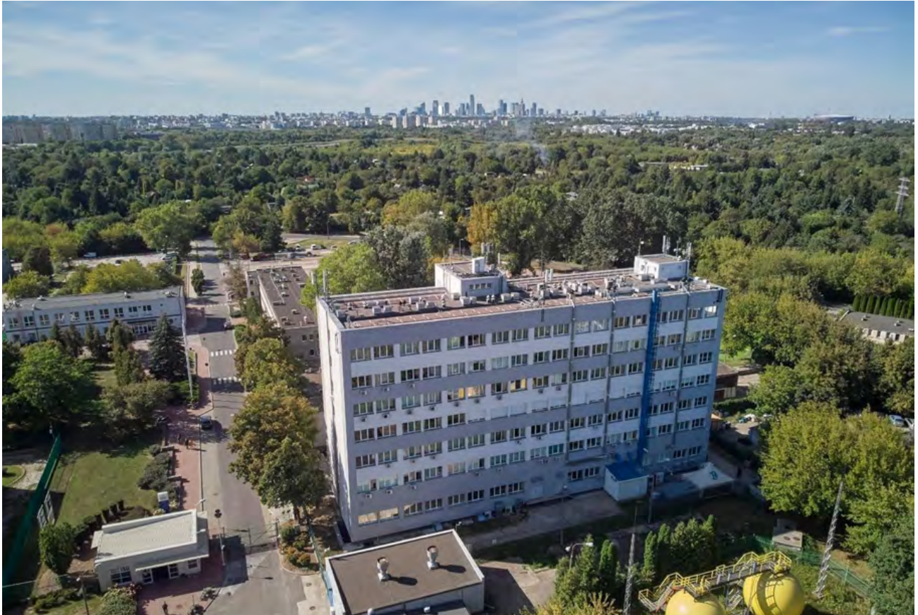
Headquarters of the Center for Hydrogen Technologies CTH2, Institute of Power Engineering – National Research Institute, Augustówka 36, Warsaw, Poland
